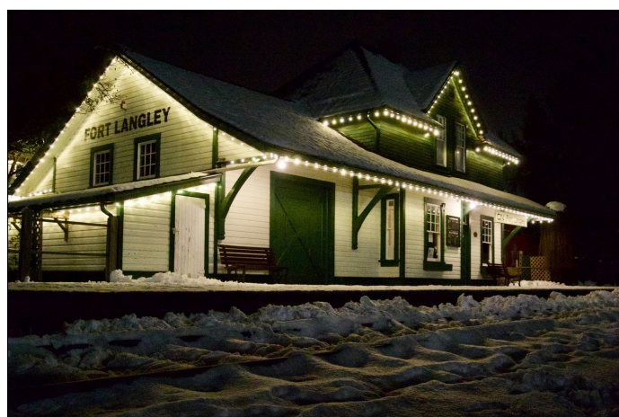
The station's new lights generously donated by Your Local Community in 2021 now turn on and off with sunset and sunrise. Many thanks to electrician and LHS member Bob McPherson for sourcing a reliable timer. Photo: Mark Forsythe
