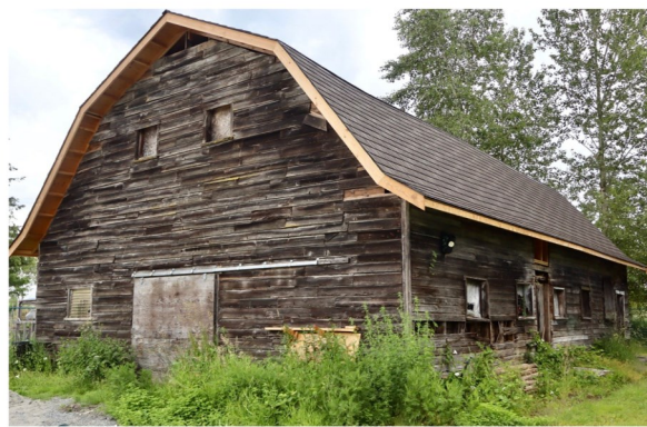
The 1915 era barn now has a new roof made from recycled tires. Photo Mark Forsythe
